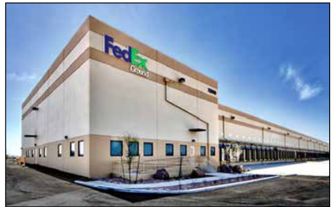
The FedEx Ground building in Sauget Business Park.
